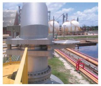
Cam-Set® DN 500 (20"), ASME 150# with spectacle plate support
